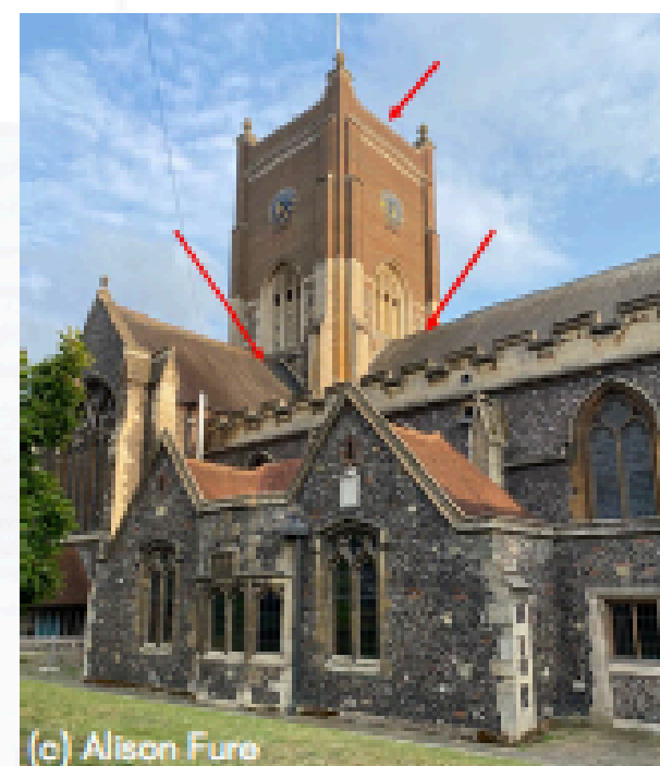
Figure 4: Photograph shows potential access points via the roof.
